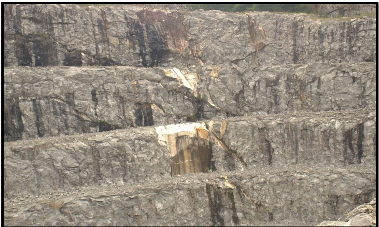
Bench System at quarry
